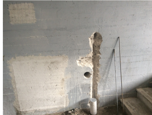
Sampling and analysis of the masonry specimens for the materials characterisation
